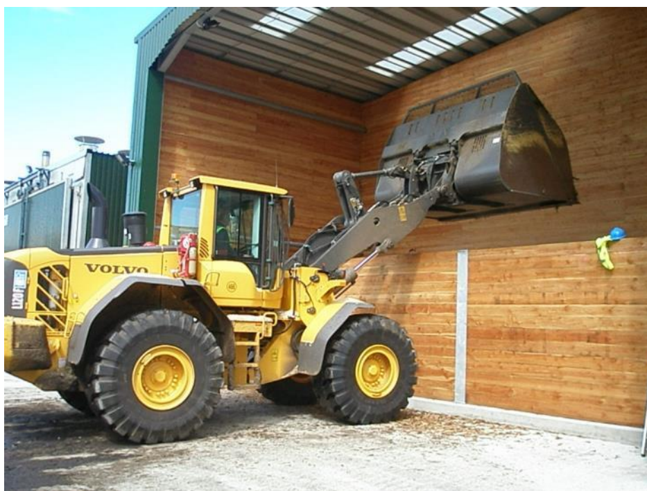
Wood Chip Delivery to Wood Chip Store for 6MW Biomass Boiler, Photo Courtesy of Sustainable Energy Ltd
